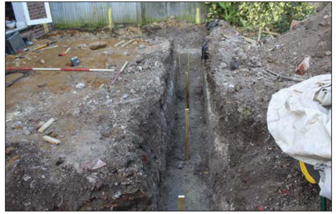
Plate 2. Footings of rear extension, looking North. Scales: 2m and 1m.
