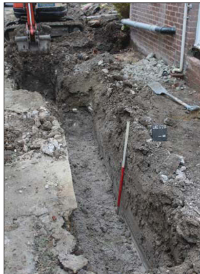
Plate 5. Footings of side extension, looking West. Scale: 1m.
