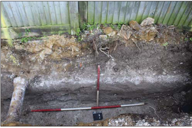
Plate 1. Footings of rear extension, looking North. Scales: 2m and 1m.
