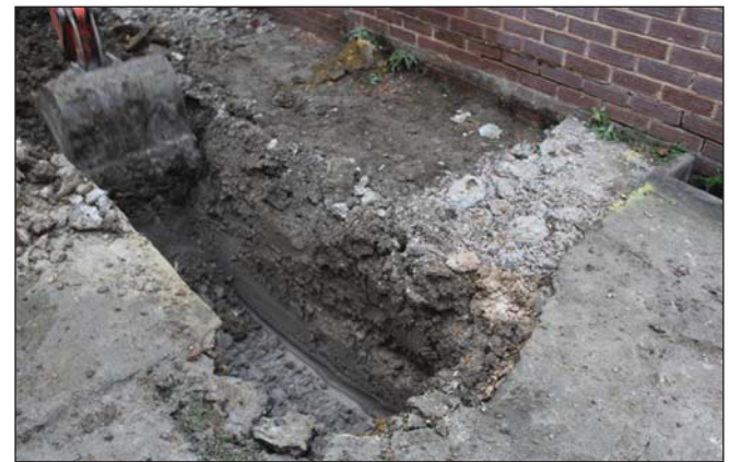
Plate 4. Footings of side extension, looking North-west.
