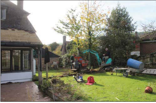
Plate 1. General view of site, looking South.
