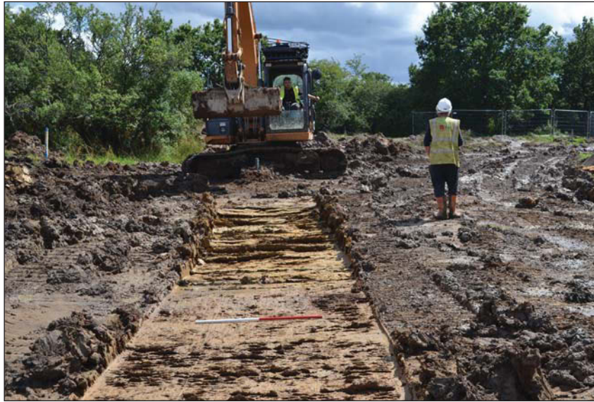
Plate 1. Overburden removed to top of natural, looking south east, Scales: 1m.
