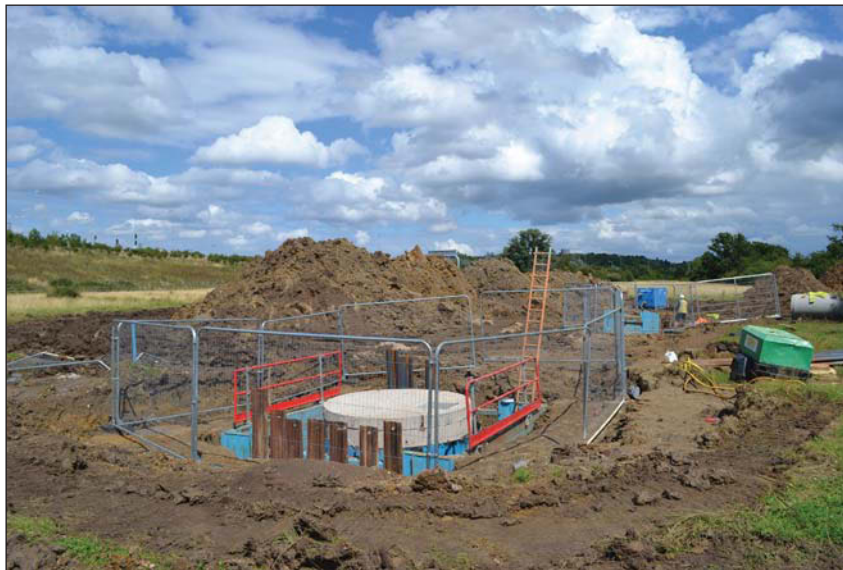
Plate 2. Location of new pumping station, looking south south east.
