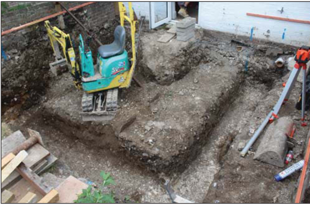
Plate 1. General shot, looking North-east.
