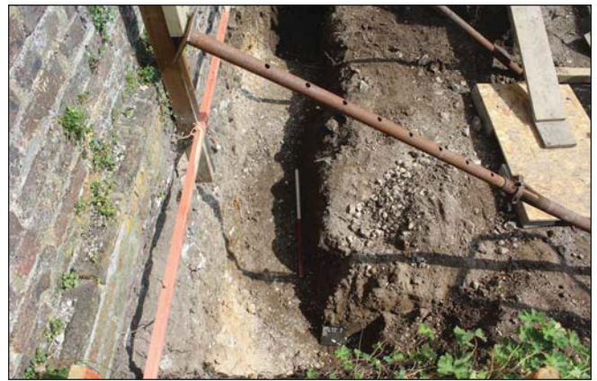
Plate 2. Pit 1, looking East. Scale: 1m.
