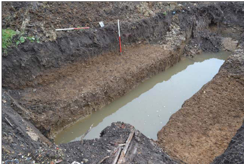
Plate 2. Trench 2 section, looking south west, Scales: horizontal 1m, vertical 1m.
