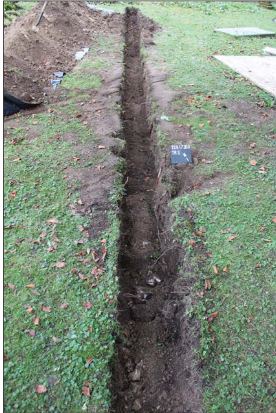
Plate 1. Trench 3, looking north-east, Scale: 0.30m.
