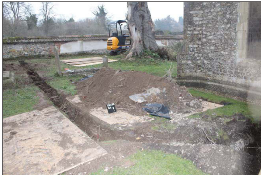
Plate 4. Trench 4, looking north-east, Scale: 0.3m.
