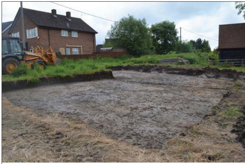
Plate 6. Plot 1, looking south west.
