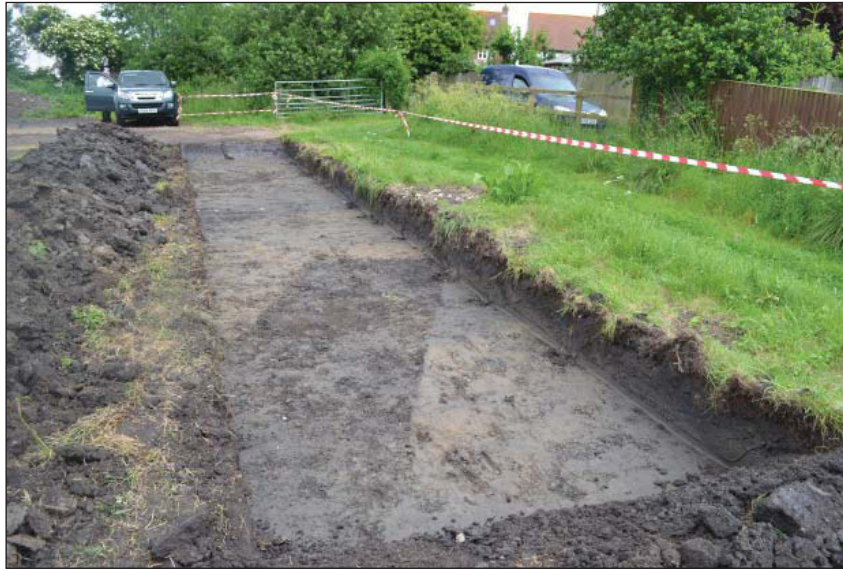
Plate 5. Access strip, looking east.
