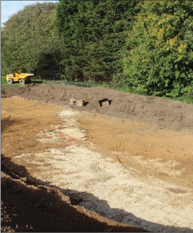
Plate 1. Excavation area, looking North-east. Scales: 2m and 1m.
