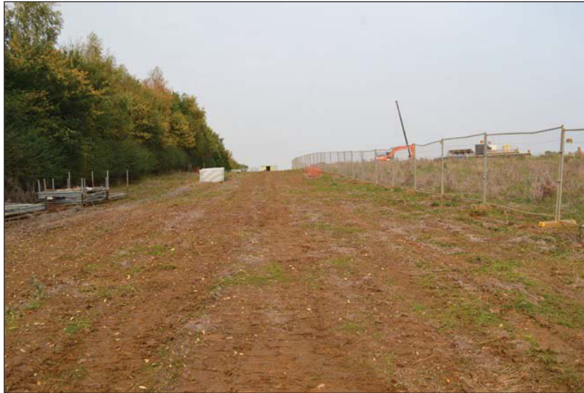
Plate 1. Pipeline route prior to stipping, looking NW.
