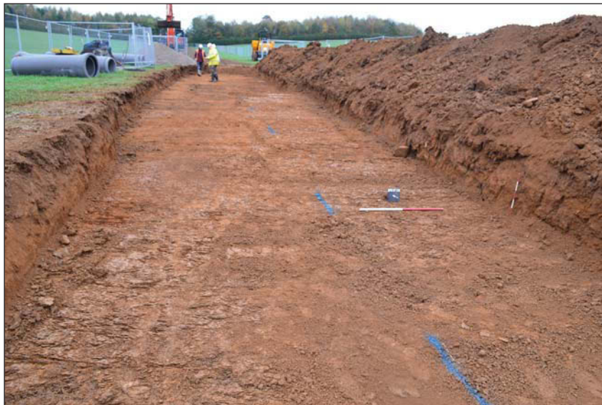
Plate 4. Route of pipeline stripped, looking NE, Scales: horizontal 1m, vertical 0.5m.
