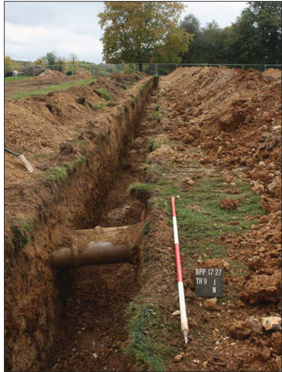
Plate 6. Trench 9, looking south, Scale: 2m.
