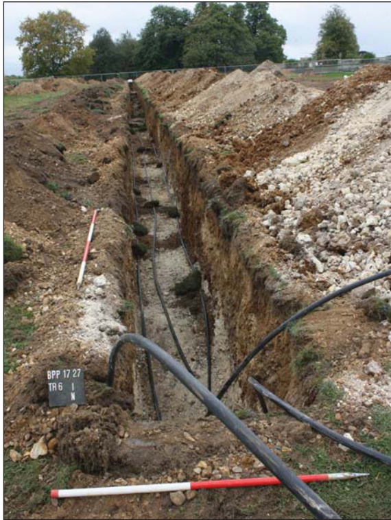
Plate 5. Trench 6, looking south, Scales: 2m and 1m.
