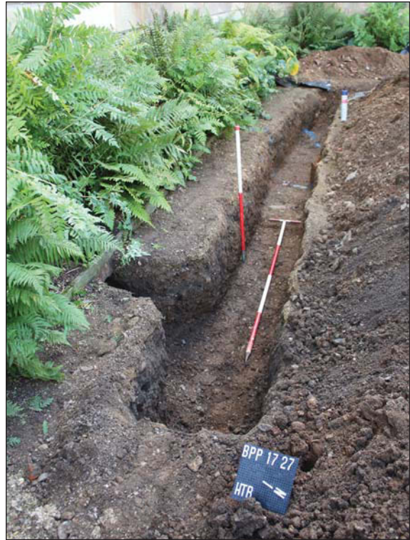
Plate 2. House trench 22 (main house), looking south-west, Scales: horizontal 2m, vertical 1m.
