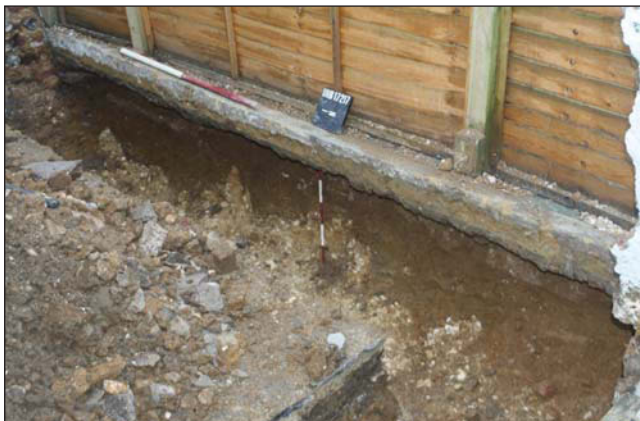
Plate 3. Western footing, looking South-west. Scale: 1m and 0.50m.
