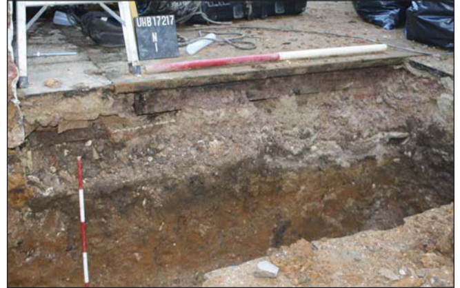
Plate 2. Northern footing, looking North-east. Scales: 1m and 0.40m.
