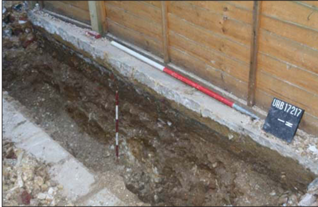
Plate 1. Western footing, looking South-west. Scale: 1m and 0.50m.
