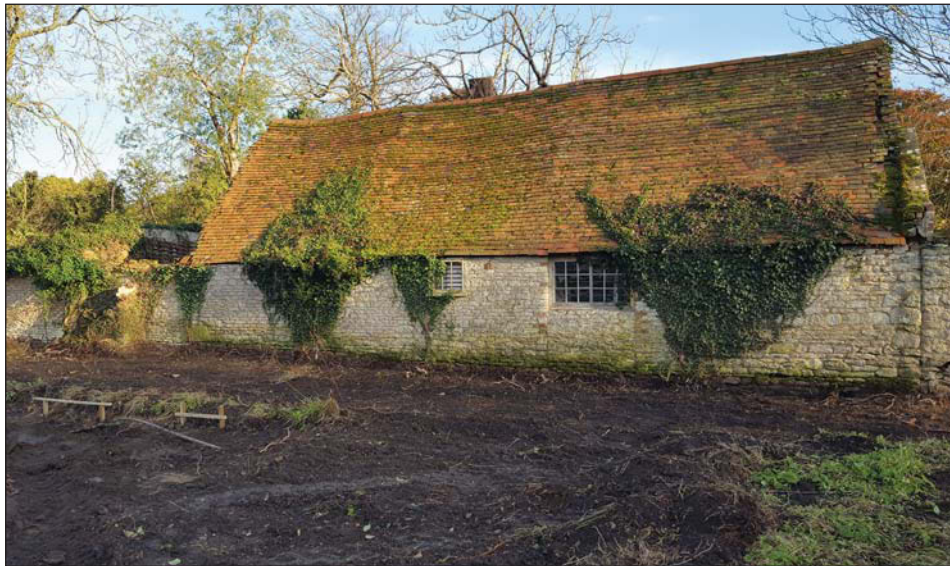
Plate 1. West elevation of adjoining Listed building, looking north east.
