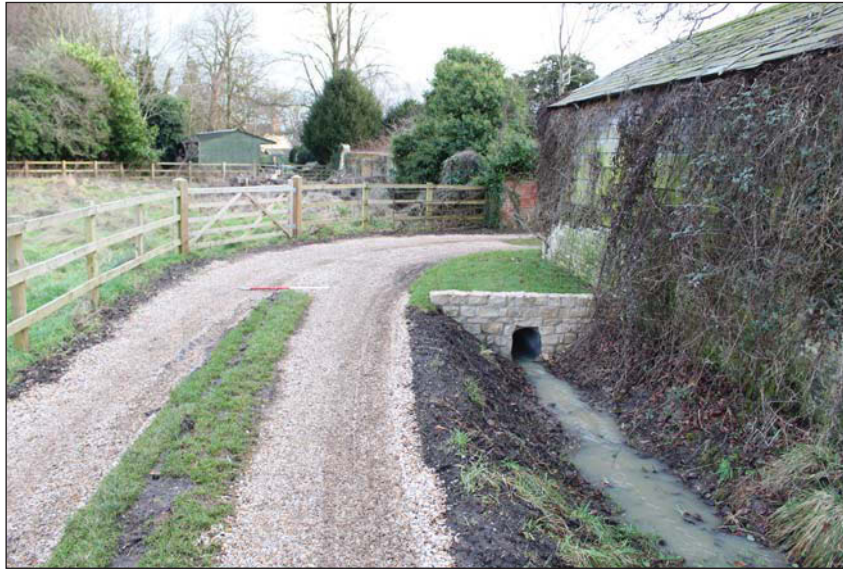
Plate 5. New access, looking south east, Scale: 1m.
