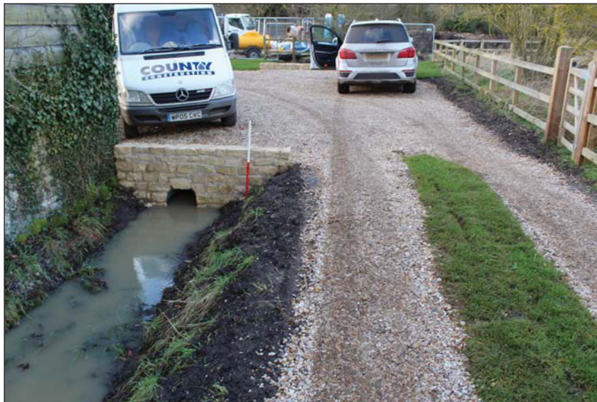
Plate 6. New access and turning circle, looking north west, Scale: 1m.
