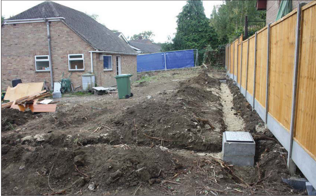
Plate 1. Drainage run around north of site, looking west.
