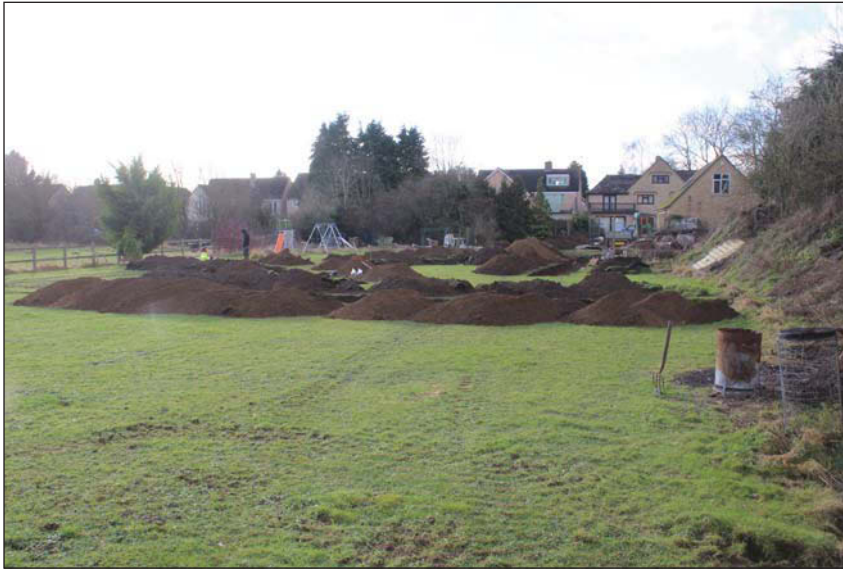
Plate 1. Area of trenching, looking southwest.
