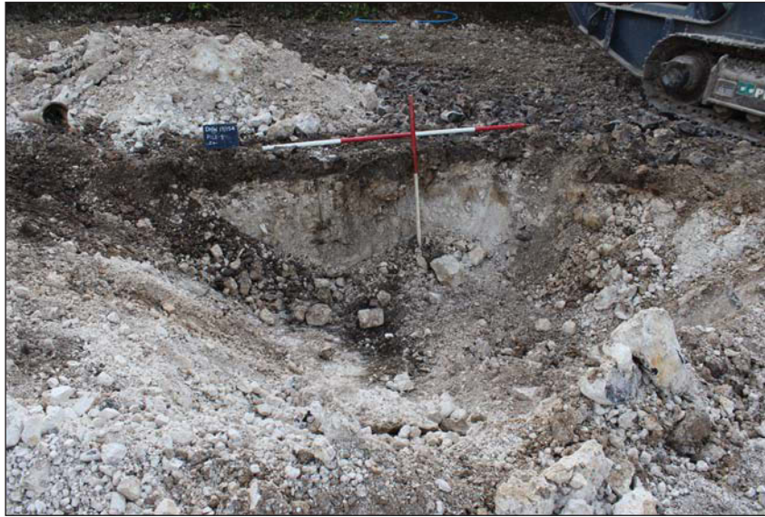
Plate 1. section of hole created removing pad 1, looking south east, Scales: 2m and 1m.
