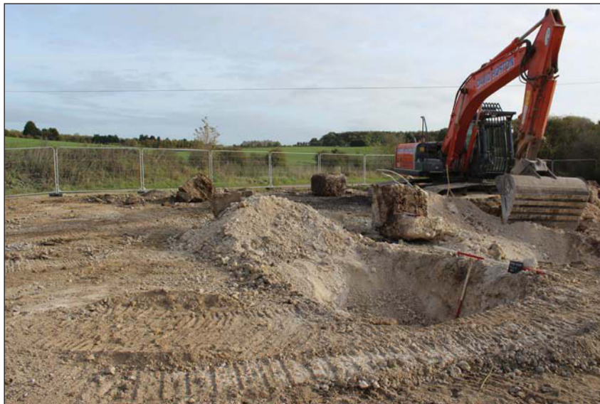
Plate 2. Pad 7 removed, looking north, Scales: 2m and 1m.
