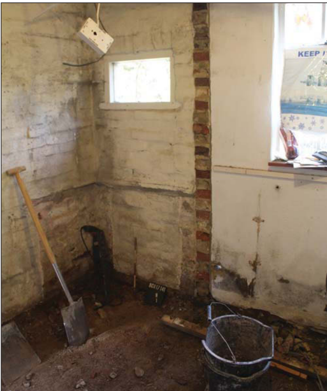
Plate 3. Rooms A and B following ground reduction, looking West. Scale: 0.50m.
