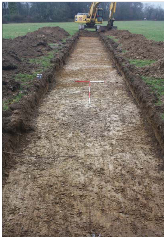
Plate 2. Trench 10, looking north east, Scales: horizontal 2m and 1m, vertical 0.3m.
