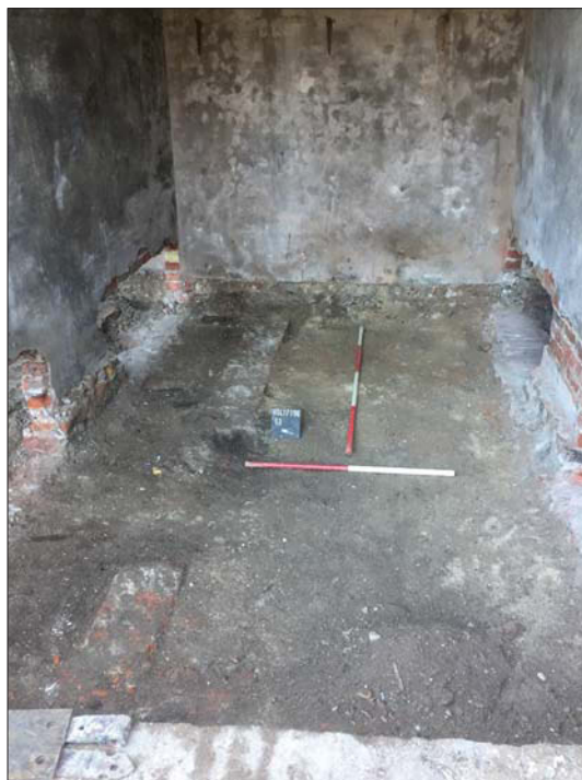
Plate 2. Walls 52, 53, 54 and 56, along with surface 55, looking East, Scales: 2m and 1m.
