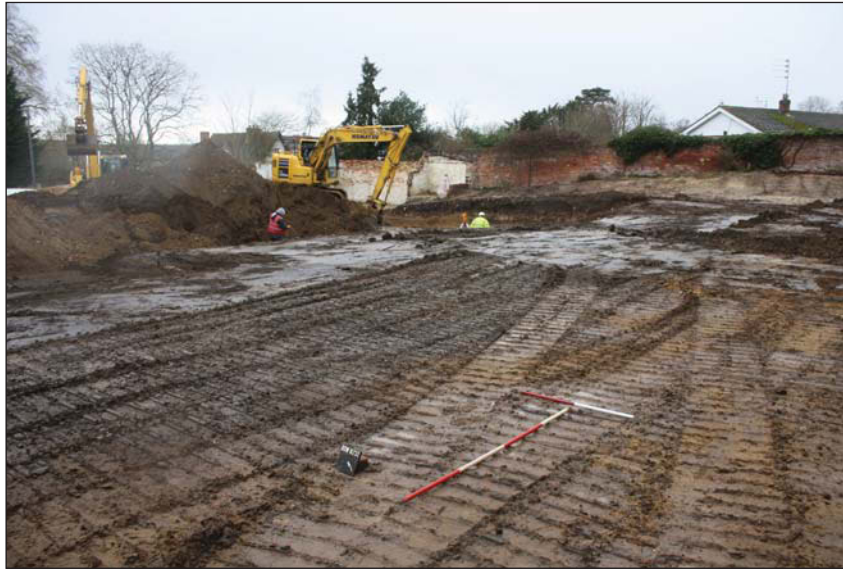
Plate 1. Upper terracing, looking south west, Scales: 2m and 1m.
