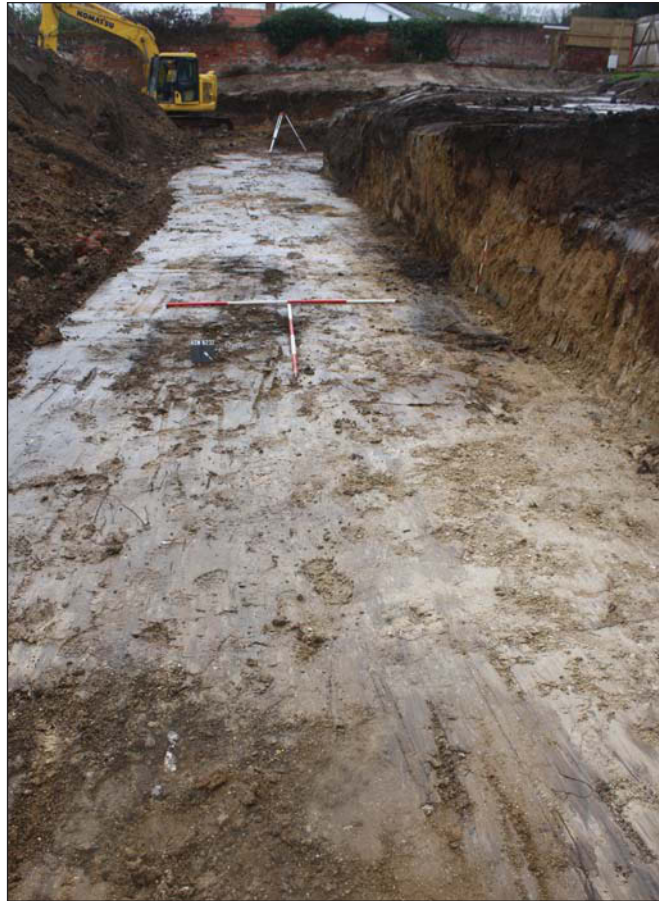
Plate 3. Lower terracing, looking north, Scales: horizontal 2m and 1m, vertical 0.5m.
