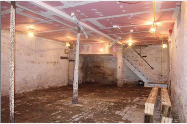
Plate 1. General view of basement, looking North-east.
