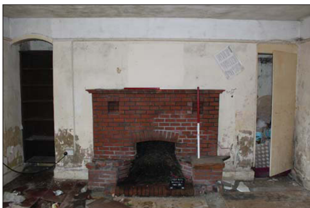
Plate 12. Old School House, Room 2, Fireplace detail, looking NE, Scales: 2 x 1m.
