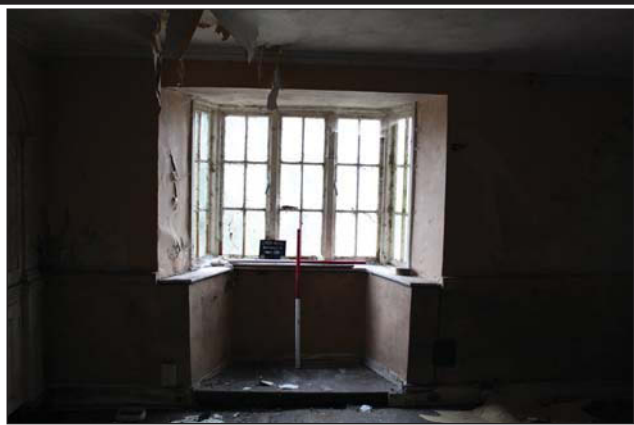
Plate 10. Old School House, Room 1, View to bay window, looking NE, Scales: 2 x 1m.
