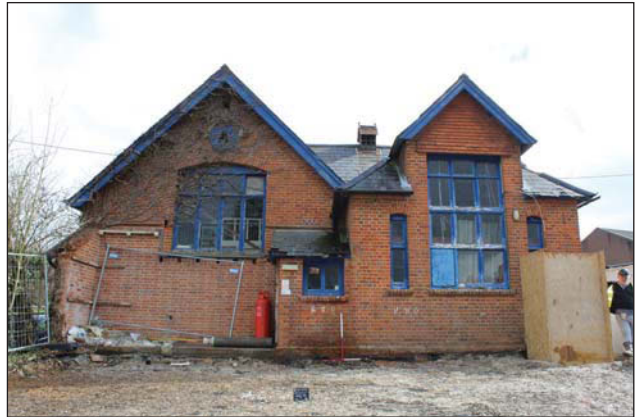
Plate 24. Former School, Northwest elevation, looking SE, Scales: 2x 1m.
