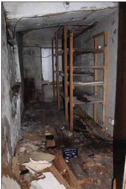
Plate 17. Old School House, Room 5, General view, looking SW.
