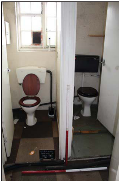
Plate 21. Old School House, Room 9, Toilets, looking SE, Scales: 2x 1m.
