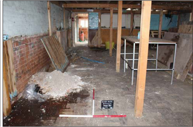
Plate 32. Former School, Room 2, General view, looking W, Scales: 2x 1m.
