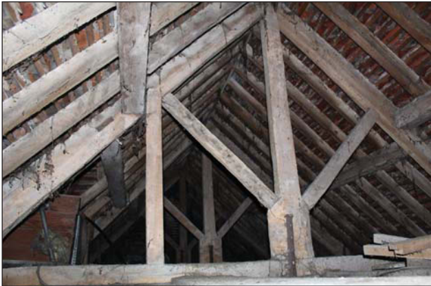
Plate 23. Old School House, loft, Roof truss detail, looking SW.
