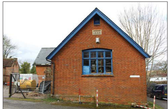
Plate 26. Former School, Southeast elevation, looking NW, Scales: 2x 1m.
