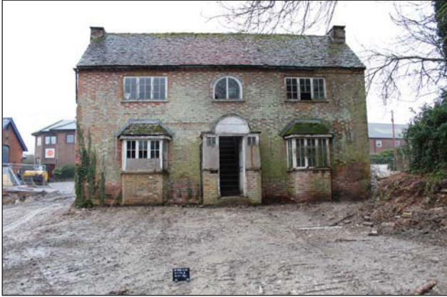
Plate 1. Old School House, Northwest elevation, looking SE.
