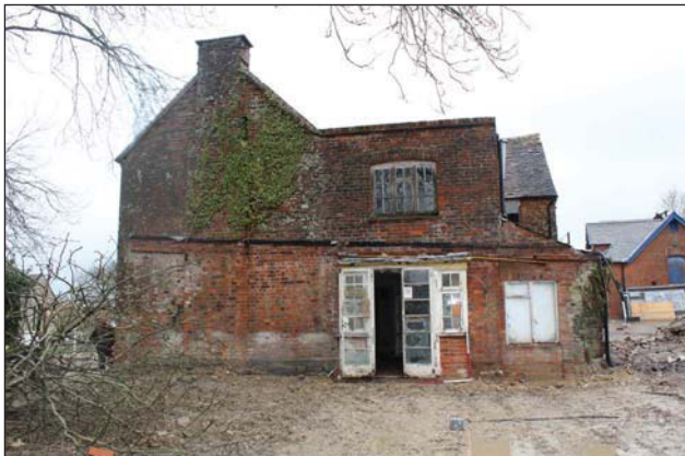
Plate 4. Old School House, Southwest elevation, looking NE, Scales: 2 x 1m.
