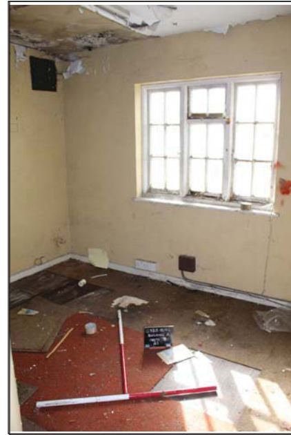
Plate 20. Old School House, Room 8, View to window, looking SE, Scales: 2x 1m.
