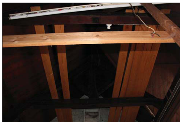
Plate 37. Former School, loft, Roof truss, looking NW.
