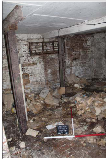
Plate 6. Old School House, Room 11, Blocked window, looking SE, Scales: 2 x 1m.
