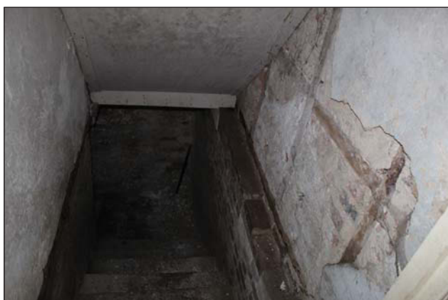
Plate 14. Old School House, Room 11, Timber box framing and cellar stairs, looking NW.
