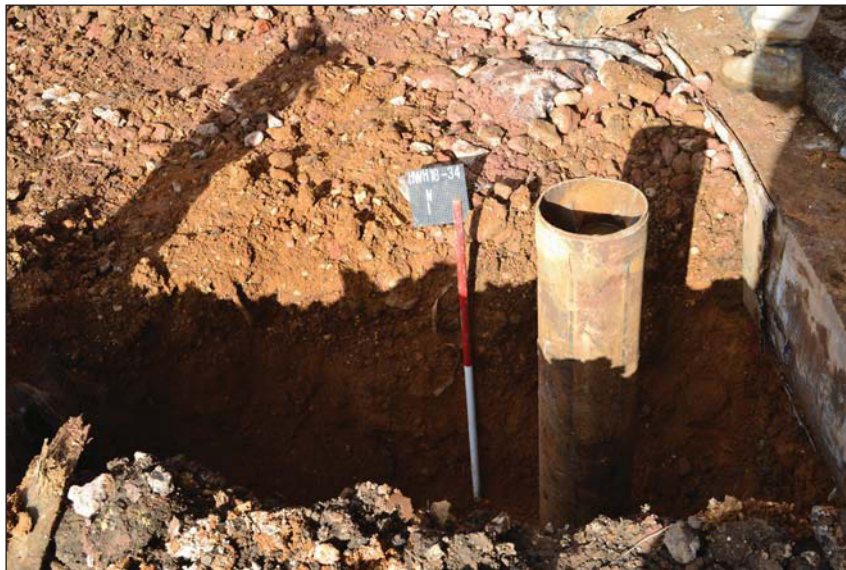
Plate 2. Garage (S), looking north, Scale: 1m.
