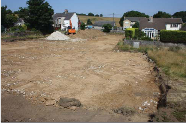
Plate 1. General view of site conditions, south of area 2, looking north.
