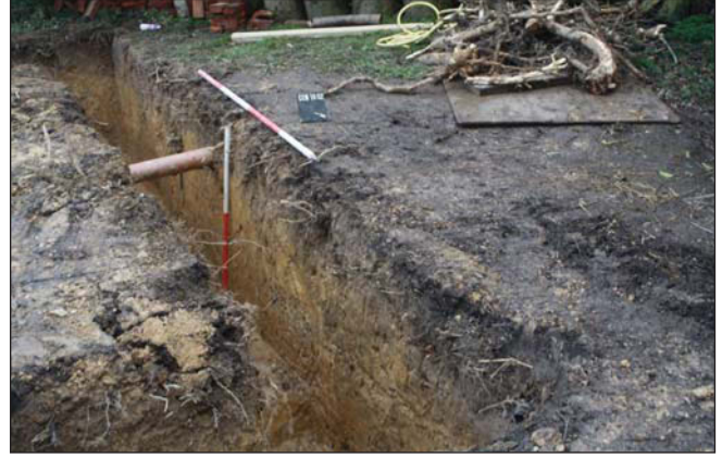
Plate 2. Footing of new studio, looking North-west. Scales: 2m and 1m.
