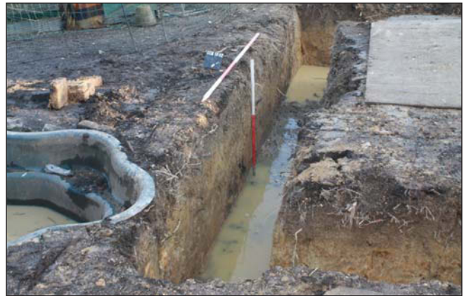
Plate 4. Footing of new studio, looking South-east. Scales: 2m and 1m.
