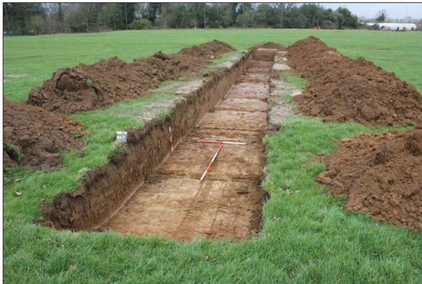
Plate 2. Trench 10, looking north north west, Scales: horizontal 2m and 1m, vertical 0.5m.
