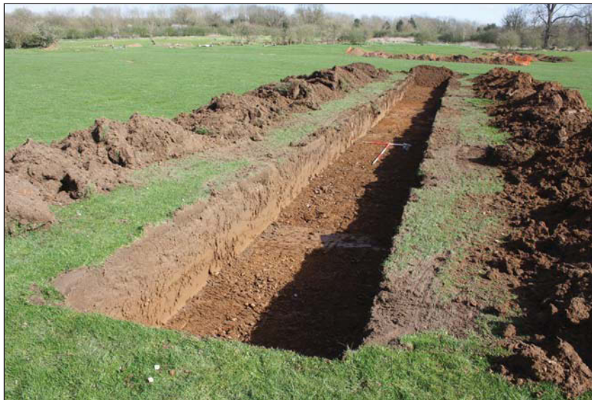
Plate 4. Trench 19, looking south east (prior to extension), Scales: horizontal 2m and 1m, vertical 0.5m.
