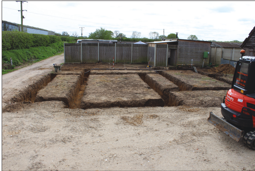
Plate 1. New footing trenches, looking south west.
