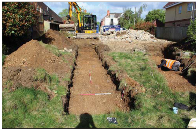
Plate 2. Trench 2 looking north west, Scales: 2m, 1m and 0.5m.
