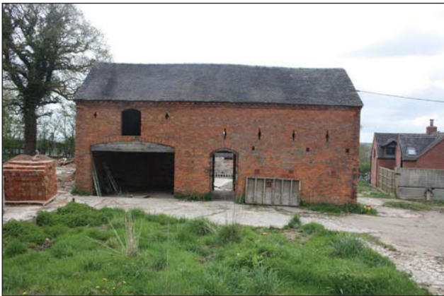
Plate 3. Barn A, exterior, west elevation looking north-east.
