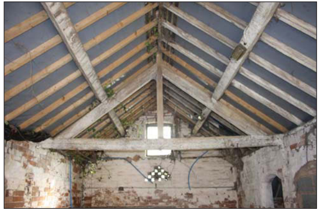
Plate 20. Barn B, interior, roof detail, looking south-east.
