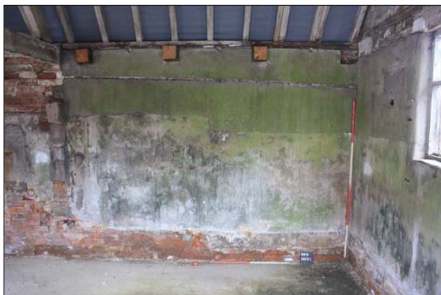
Plate 27. Barn C, interior, details of cut joists, looking north-east. Scales 2m, 1m.
