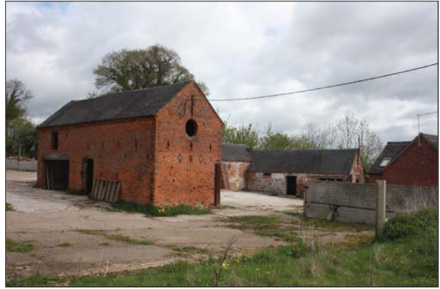
Plate 2. Barn A, exterior, south and west elevations, looking north.
