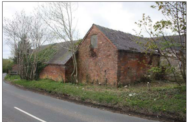
Plate 22. Barns B and C, exterior, north and east elevations, looking south.
