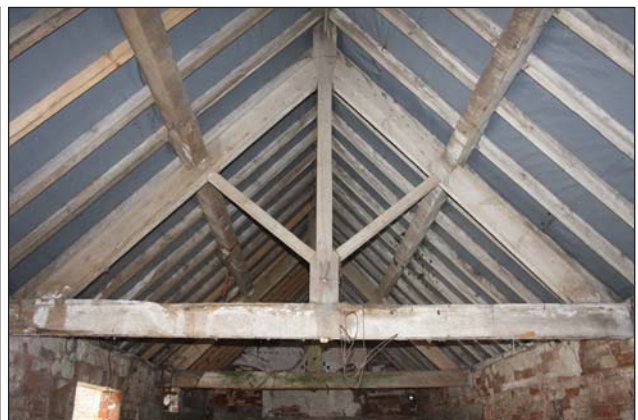
Plate 28. Barn C, interior, roof truss detail, looking north-west.
