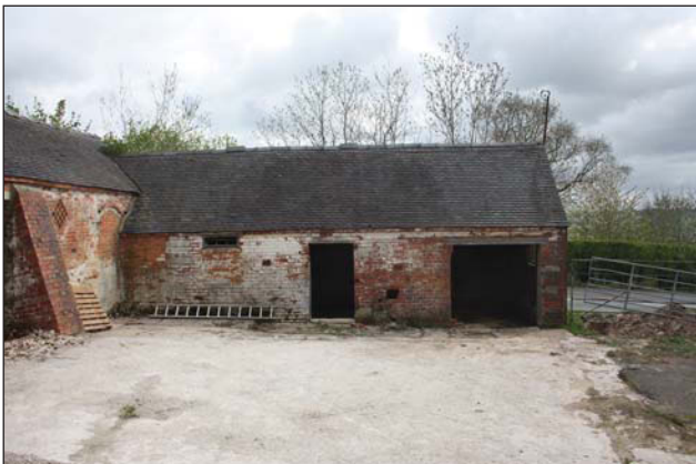
Plate 21. Barn C, exterior, west elevation, looking north-east from courtyard.
