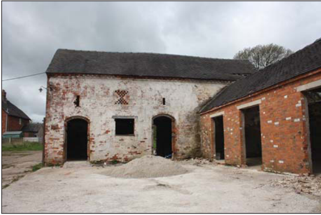
Plate 1. Barn A, exterior, looking east from courtyard.
