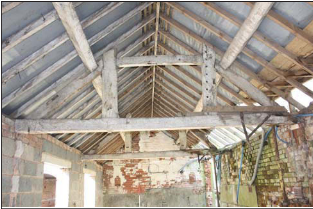
Plate 19. Barn B, interior, roof truss detail, looking south-west.
