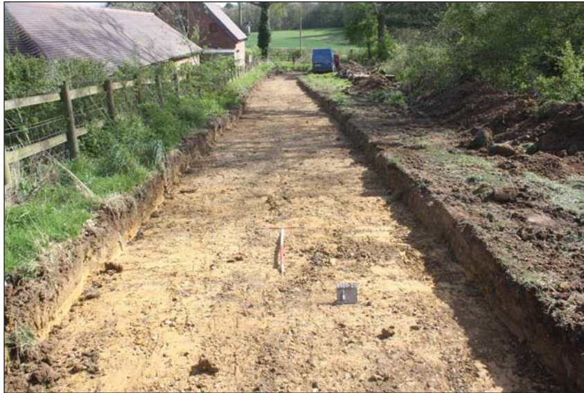
Plate 1. Reduced dig at southern end, looking south, Scales: 1m and 0.5m.
