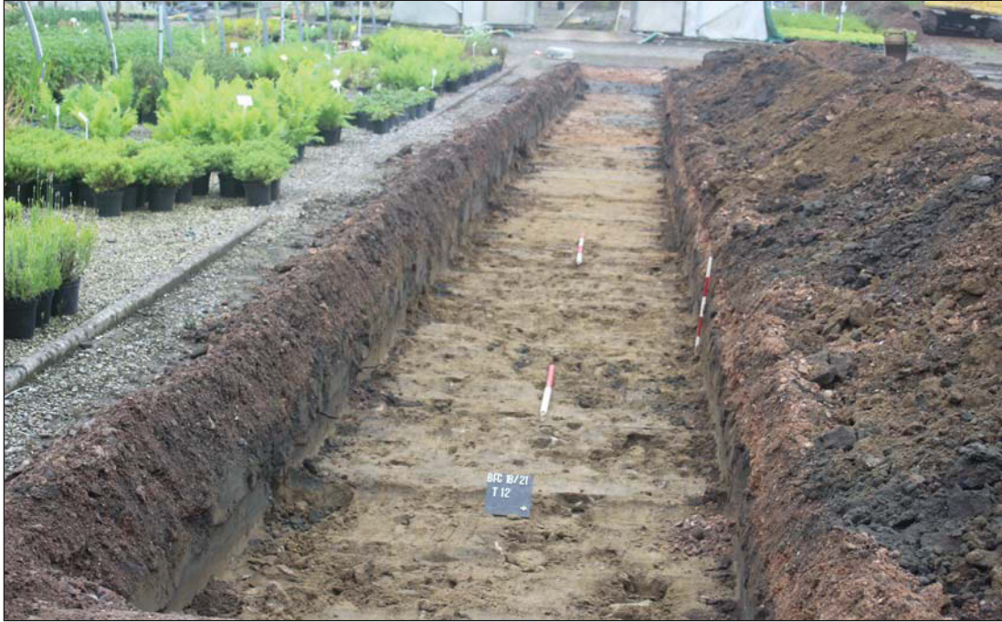
Plate 5. Trench 12, looking west, Scales: 2m, 1m and 0.5m.
