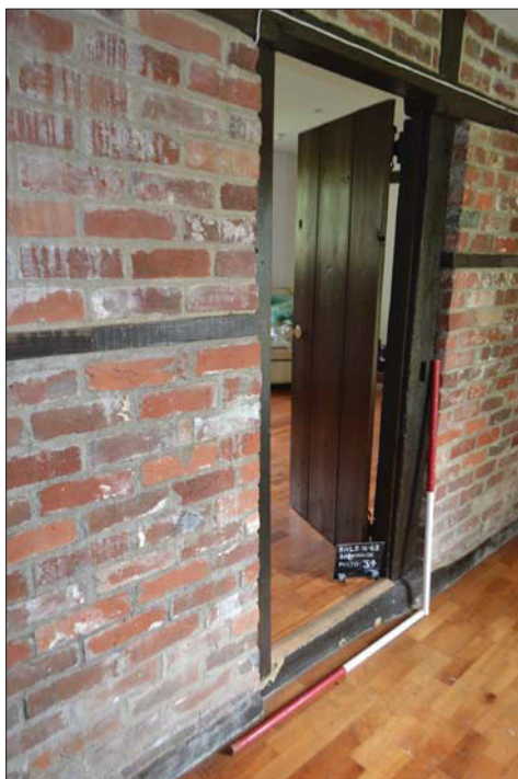
Plate 35. Corridor, timber detail, Scales: 1m.
