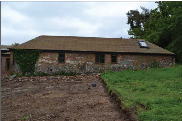
Plate 31. Block B, north-west elevation, looking south-east, Scales: 1m.
