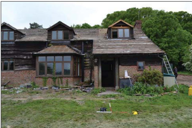
Plate 3. Front elevation, north-west end, looking south-west.
