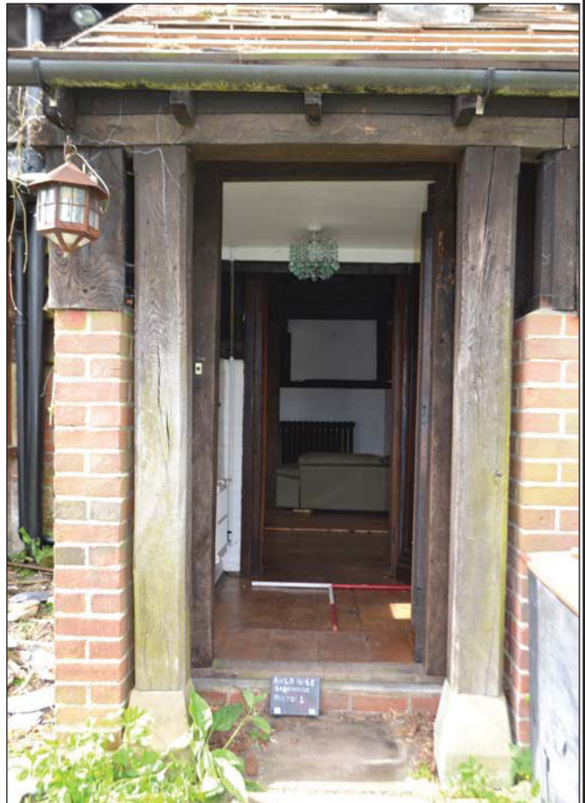
Plate 4. Entrance hall, looking south-west. Scales: 1m.
