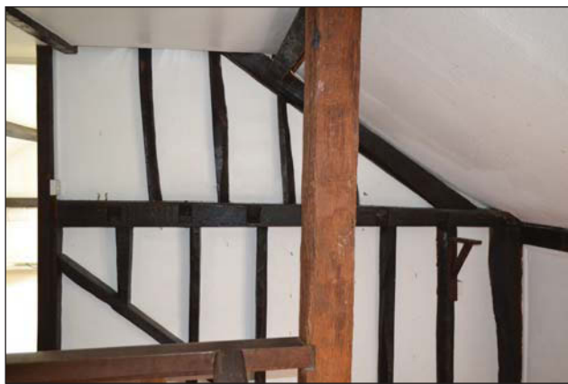
Plate 19. Hallway timber detail, looking south-east.
