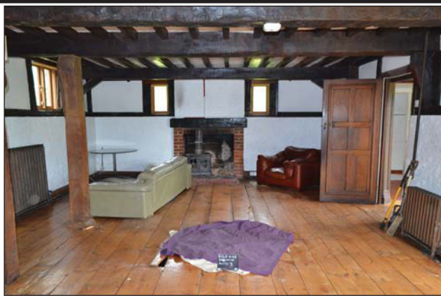
Plate 11. Room 2, looking north-west, Scales: 1m.
