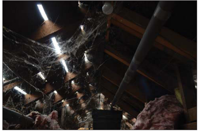
Plate 28. Block A, roof detail, looking south-east.
