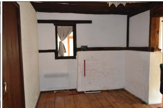
Plate 16. Room 8 wall detail, looking south-east, Scales: 1m.
