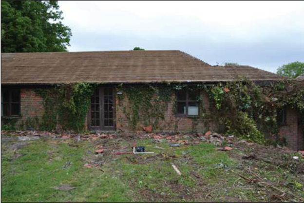
Plate 29. Block B, south-east elevation looking north-west, Scales: 1m.
