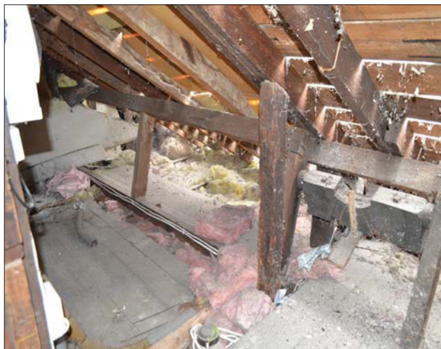
Plate 26. Room 13, roof detail, looking north-west.
