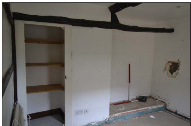
Plate 36. Room 4, looking west, Scales: 1m.
