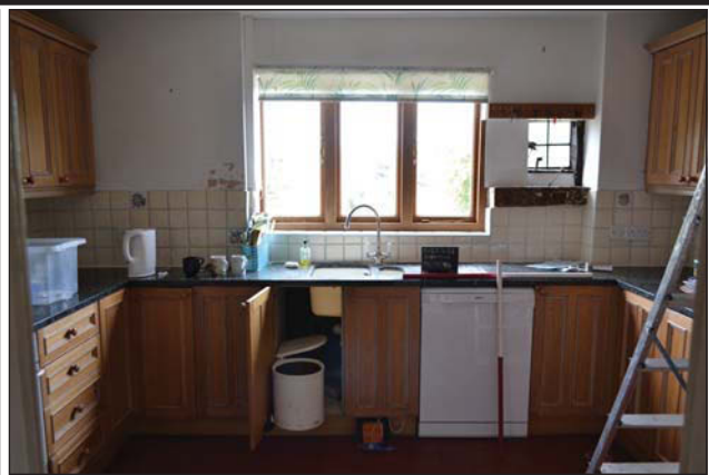
Plate 18. Room 9, looking north-east, Scales: 1m.
