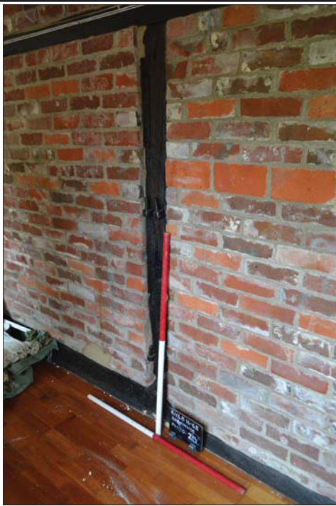
Plate 33. Corridor, timber detail, Scales: 1m.
