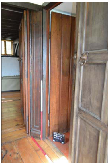
Plate 9. Timber detail, entrance hall, looking west, Scales: 1m.
