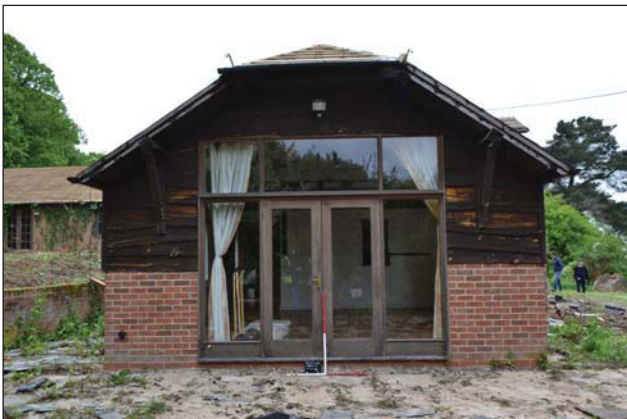
Plate 39. Block C gable end, looking north-west, Scales: 1m.
