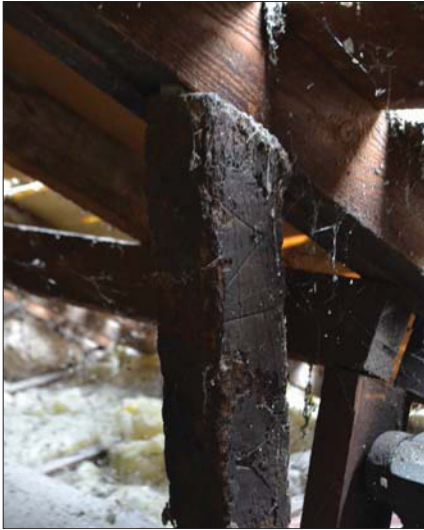
Plate 27. Room 13, carpenter's mark.
