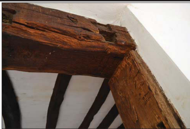
Plate 17. Room 8, carpenter's mark.
