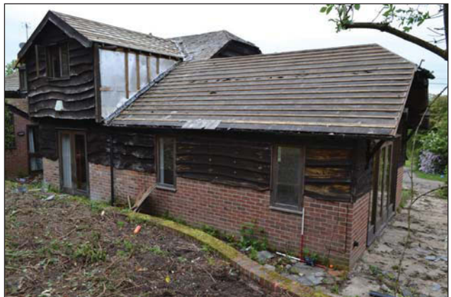
Plate 40. Block C, rear, looking north, Scales: 1m.
