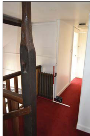
Plate 20. Hallway timber detail, looking north-west, Scales: 1m.
