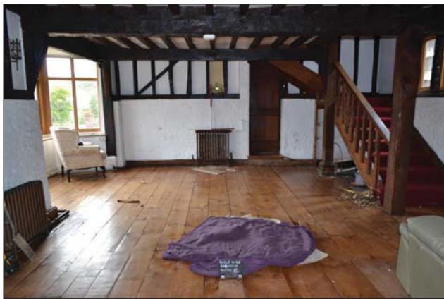
Plate 13. Room 2, looking south-east, Scales: 1m.
