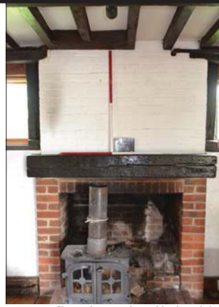
Plate 12. Room 2, fireplace detail, looking north-west, Scales: 1m.
