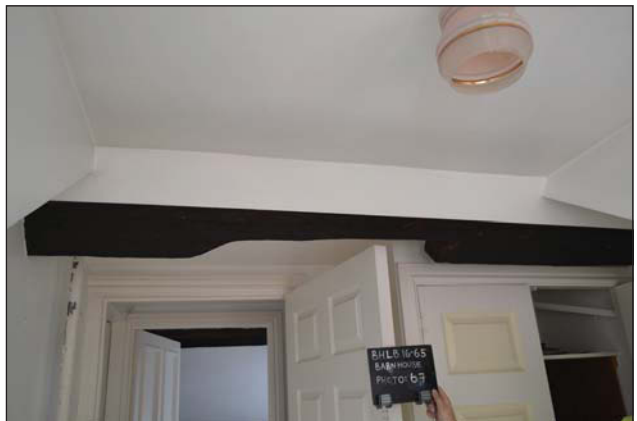
Plate 22. Room 14, purlin detail.
