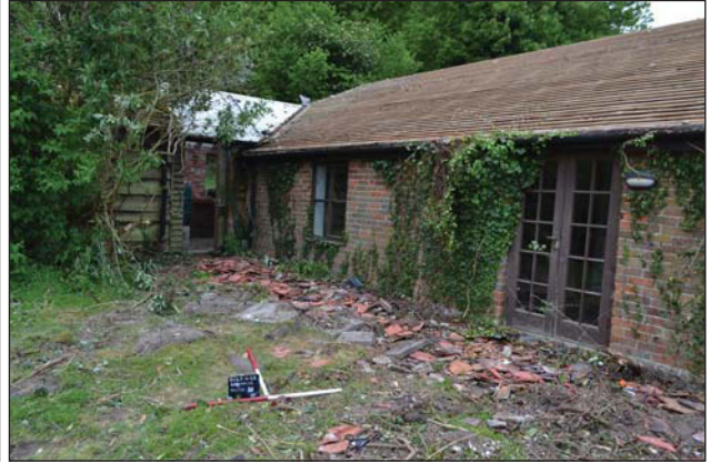
Plate 44. Blocks B and D oblique, looking west, Scales: 1m.
