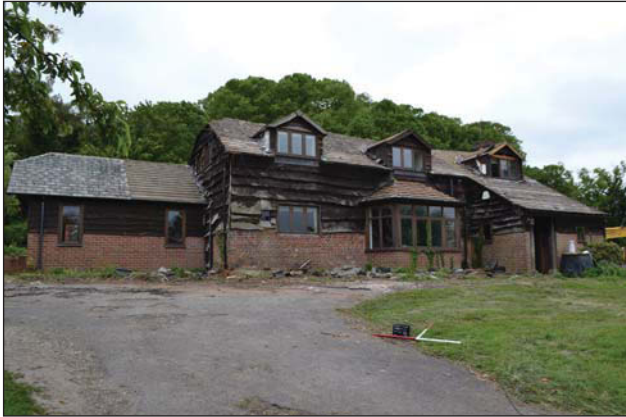
Plate 1. Exterior, general view, front, looking west.
