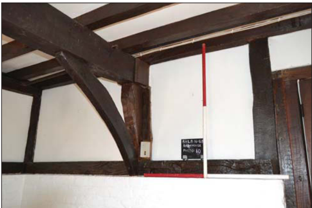
Plate 15. Room 2, timber detail, looking north-east, Scales: 1m.
