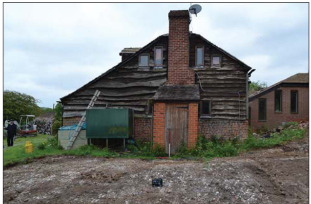
Plate 8. Block A gable, looking south-east, Scales: 1m.
