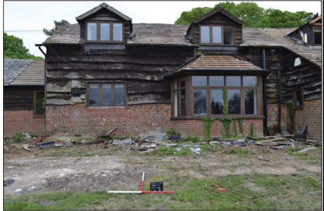
Plate 2. Front elevation, centre, looking south-west.
