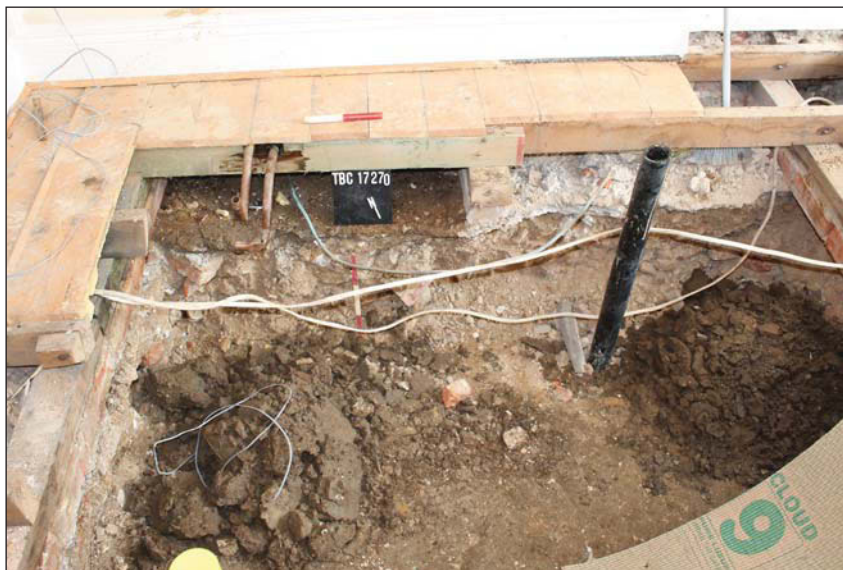
Plate 4. Rubble fill excavated in Dining Room floor, looking north west, Scales: 0.2m and 0.3m.
