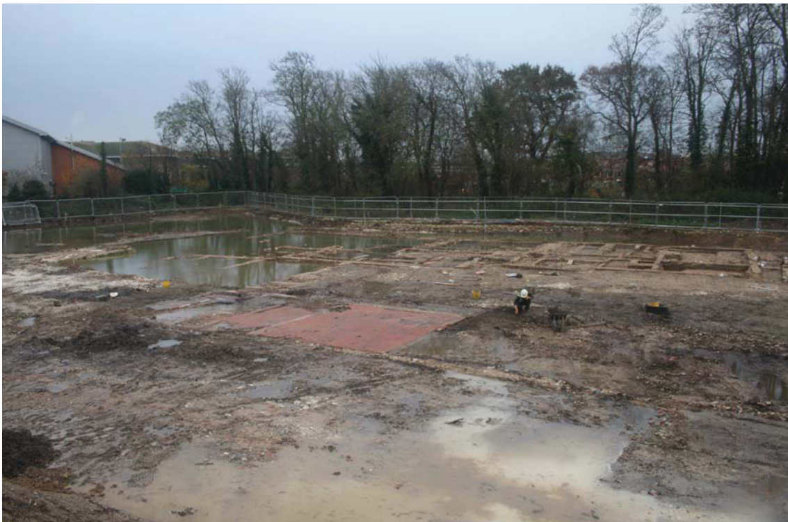
Plate 2. Excavation conditions, looking south-east.
