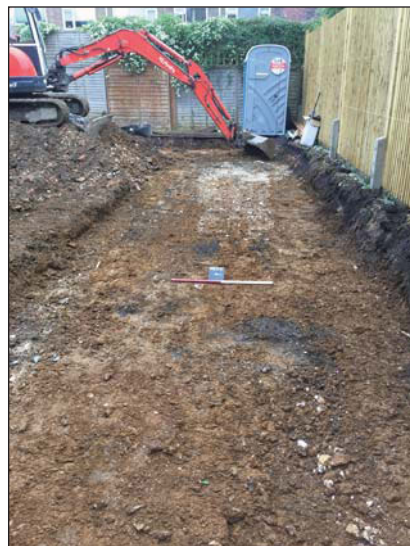
Plate 5. General view of southern part of site, looking East. Scale: 1m.
