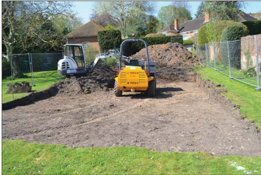
Plate 1. Ground reduction in progress, looking north.
