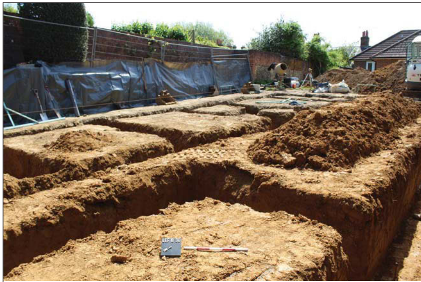
Plate 2. Excavated footings, looking south east, Scales: 0.5m.
