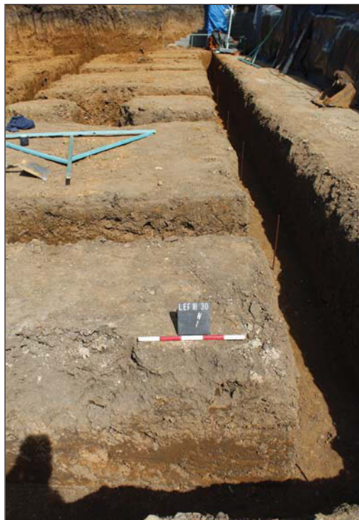
Plate 4. Excavated footings, looking north, Scales: 0.5m.
