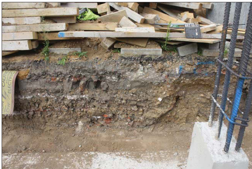
Plate 4. Exposed section under Heath road, eastern section, looking south.
