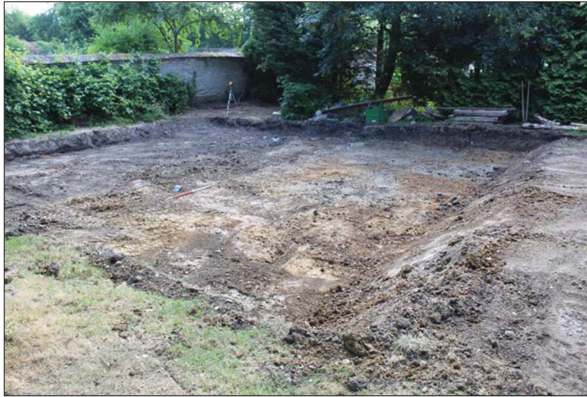
Plate 1. Area of ground reduction, looking north east, Scales: 1m and 0.2m.
