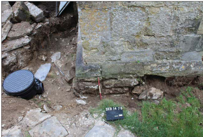
Plate 2. South-east corner buttress foundation of 13th-century chancel, looking west, Scale: 0.3m.
