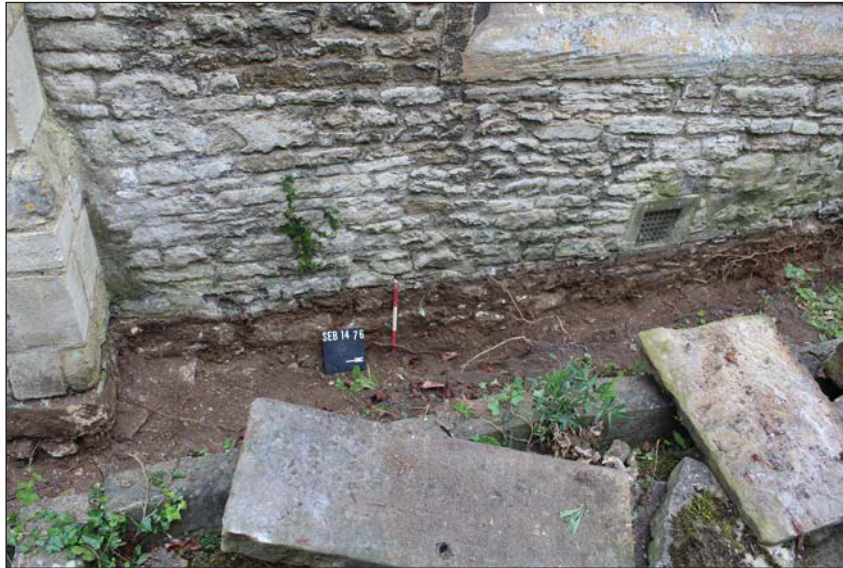
Plate 3. East Sacristy wall foundation, looking west-north-west, Scale: 0.3m.
