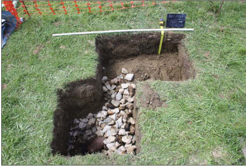
Plate 1. Existing soakaway with pipe, looking west, Scales: 1m.
