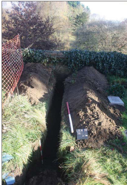
Plate 2. New drainage and soakaway, looking east, Scales: 1m and 0.5m.
