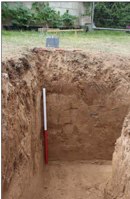
Plate 2. Section of the footings, looking west, Scales: 1m and 0.5m.
