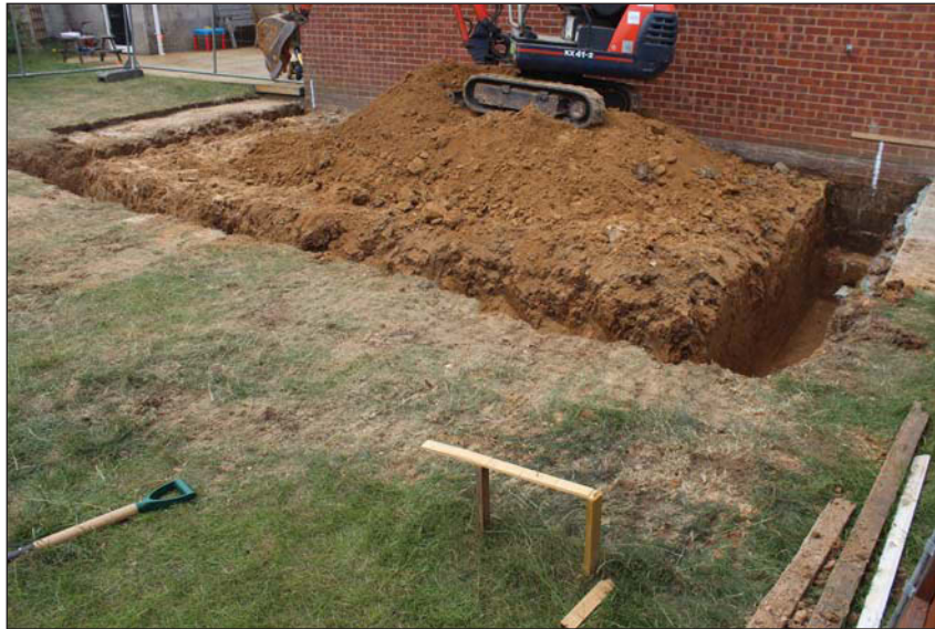
Plate 1. Excavated footings, looking north west.
