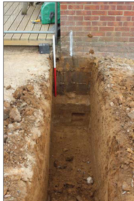
Plate 3. Existing footings, looking north, Scale: 1m.
