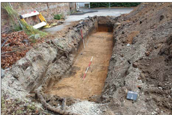
Plate 5. Trench 3 Looking south, Scales: 2m and 1m.
