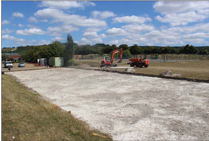
Plate 1. Reduced area in north east, looking south east.
