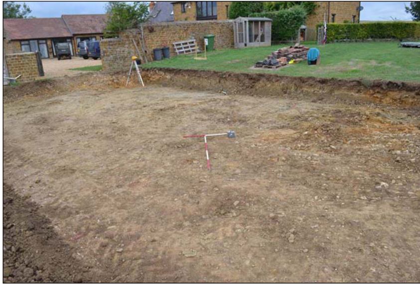
Plate 1. Final reduction on area, looking north west, Scales: 2m and 1m.
