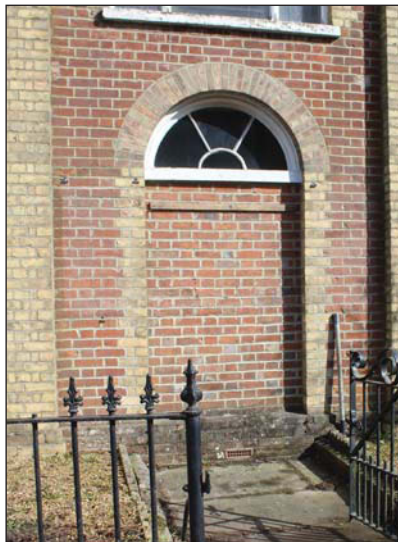
Plate 5. Original front door (now blocked), looking East North-east.
