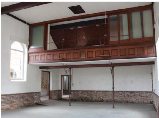
Plate 13. Worship area D, looking North.
