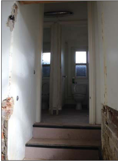
Plate 19. Room F, looking North-east from room C.
