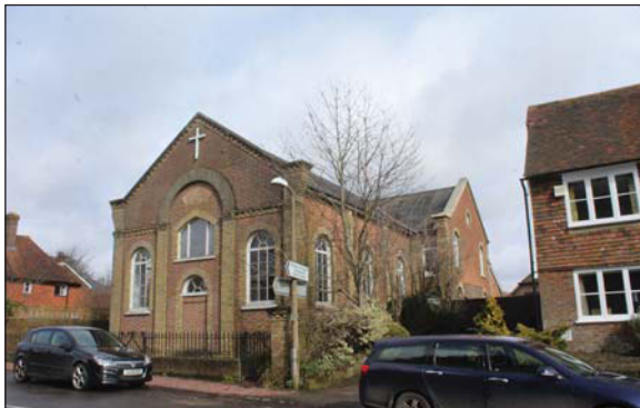
Plate 3. General view, looking North.
