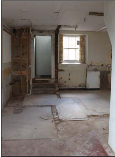
Plate 11. Room C, looking North-east from entrance lobby A.
