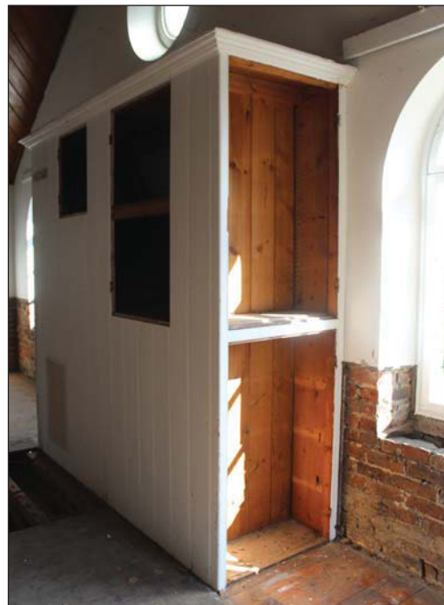
Plate 25. Wooden surround of staircase J, looking East.
