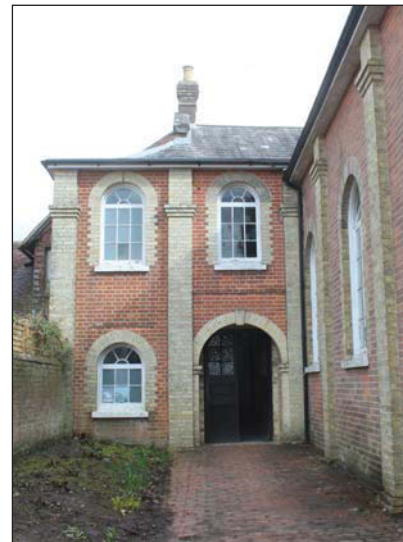
Plate 6. Present main entrance, looking North-east.
