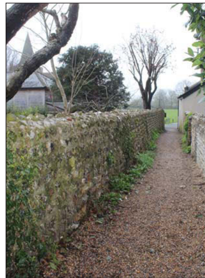
Plate 4. West side of wall, looking South South-east.
