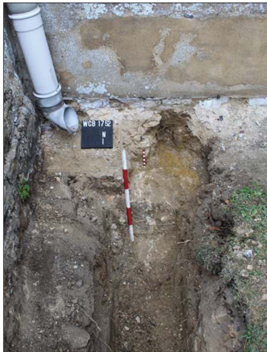
Plate 4. The overlying 15th century foundation, with a lower foundation course beneath.
