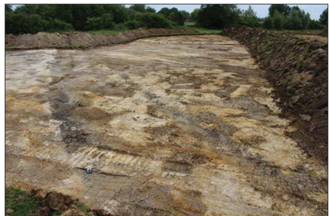
Plate 4. Cell 3, looking North East
