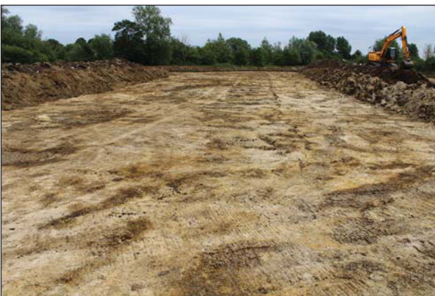
Plate 3. Cell 2, looking North East
