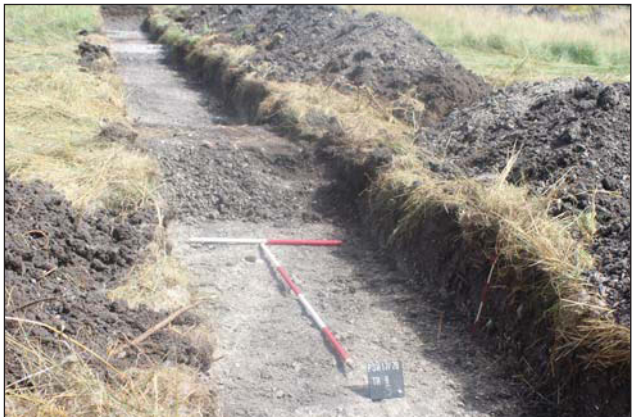
Plate 4. Trench 8, looking E, Scales: 2m, 1m and 0.5m.
