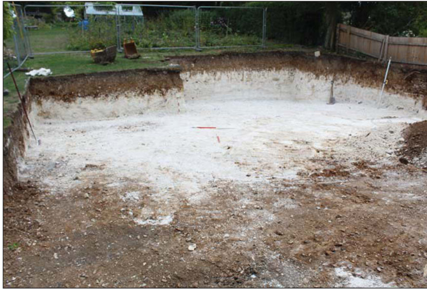
Plate 3. Full depth excavation, looking north north east, Scales: 2m and 1m.
