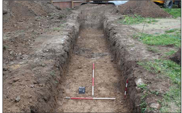
Plate 2. Trench 2, looking South. Scales: 2m, 1m and 0.50m.
